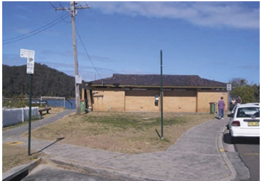
Existing amenity building at the end of Picnic Parade
